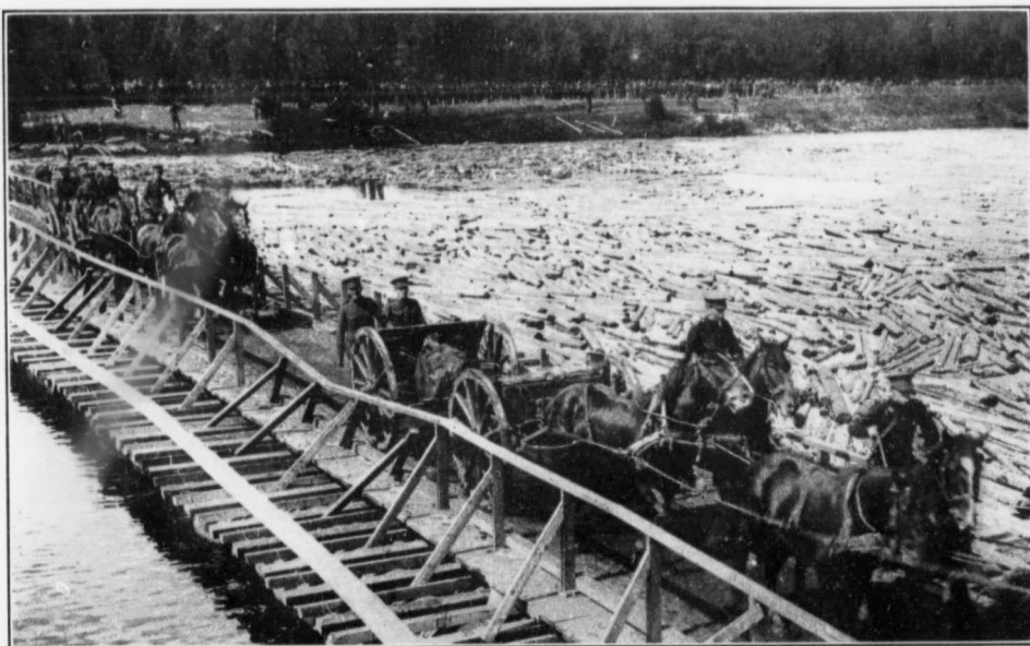
ARTILLERY USING PONTOON BRIDGE. The Artillery are here seen crossing pontoon bridge over Jacques Cartier River at Valcartier.
