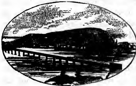
MONTREAL AND VICTORIA BRIDGE.
