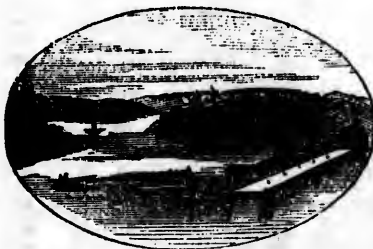
ENTRANCE TO CORNWALL CANAL.
