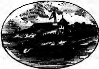
FORT HENRY — MARTELLO TOWER CEDAR ISLAND.
