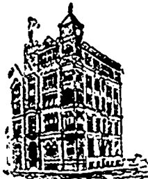
HEAD OFFICE BUILDING, MONTREAL.
