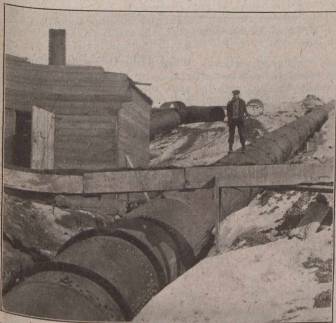
FIG. 1—EUGENIA FALLS PENSTOCK, 54-INS. DIAMETER, WITH TRIPLE-RIVETED BUTT JOINT ON LONGITUDINAL SEAM AND DOUBLE-RIVETED LAP ON GIRTH SEAM
