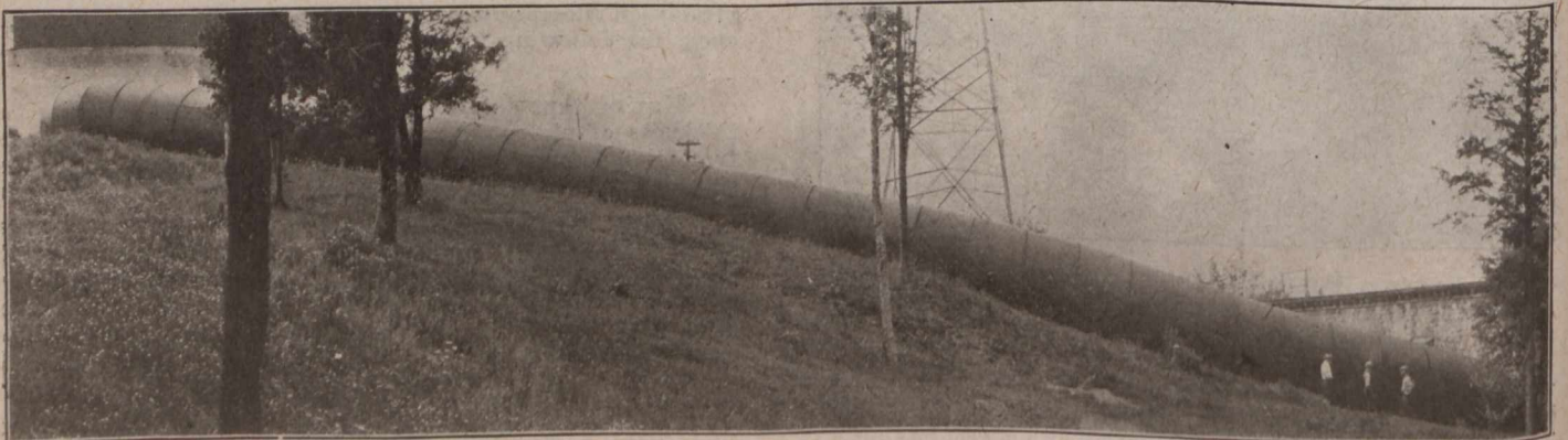
FIG. 4—PENSTOCK, 10-FT. DIAMETER, WITH SINGLE-RIVETED LAP JOINTS (AT HANNAWA FALLS, N.Y.)
