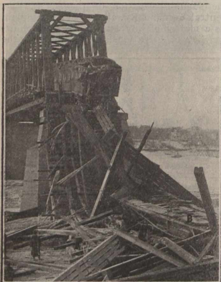
Wreckage of the Timber Truss.
