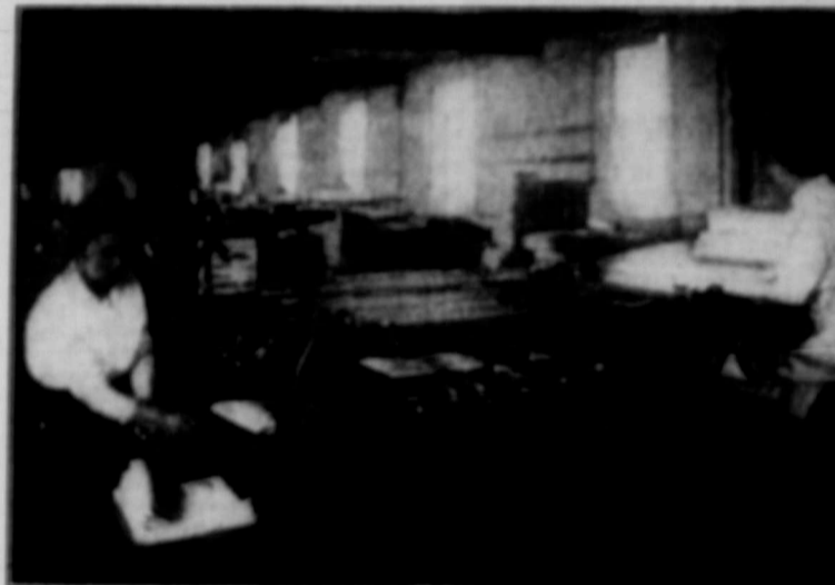
One of the big folding machines. Large eight-page sheets are placed in this machine, which automatically folds them twice and throws them out in a pile.
