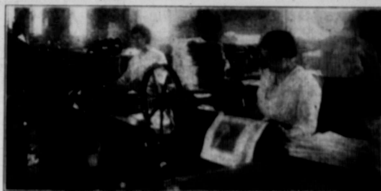
After the various sections of The Guide are gathered in proper order in the bindery then they go to the stitching machine, as shown in this picture, where the little wire stitches are placed in the back to hold the pages together. These stitchers, like all other machinery in The Guide plant, are operated by electricity.
