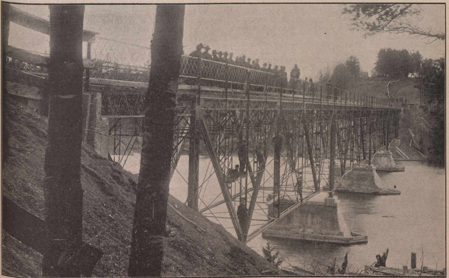
MADAWASKA BRIDGE: NEAR ARNPRIOR.
