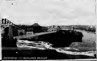
DISPERSED AND CHATELAIN BRIDGES
