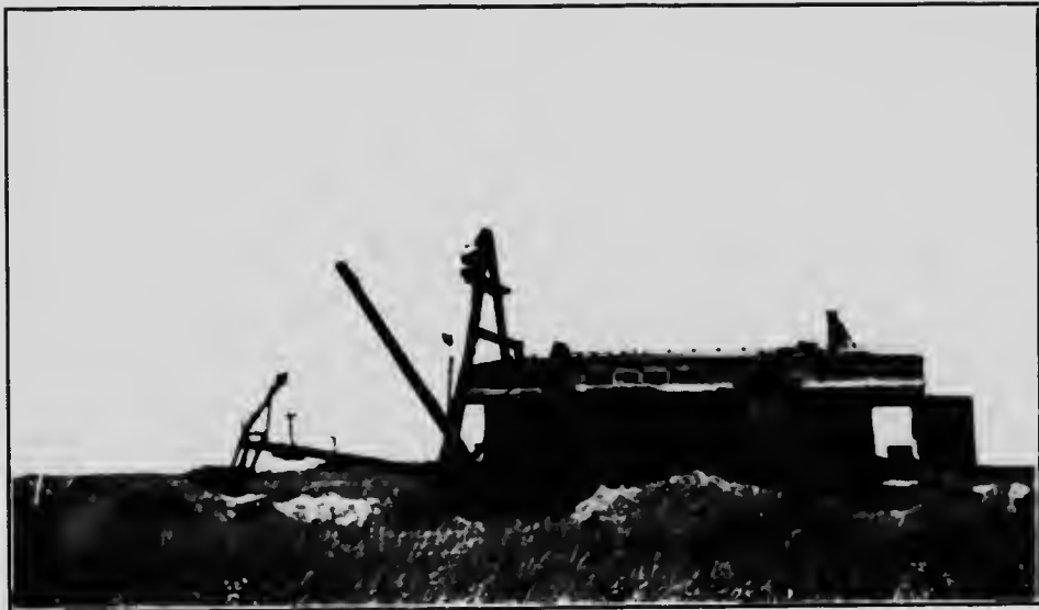
Plate 8.—Walking Dredge at Work on Open Muskeg. (Tp. 4, Rge. 7, east of Principal Meridian.)
