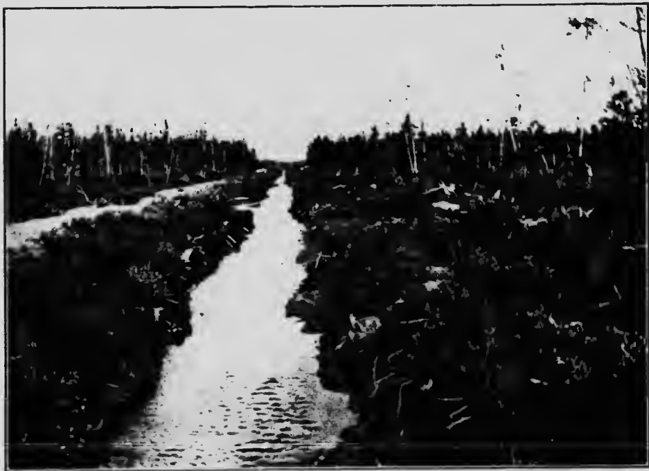
Plate 9.—Ditch Dug by Walking Dredge, Showing Road Alongside Made with Earth Removed.
