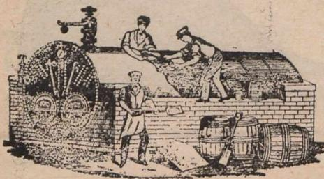
For COATING BOILERS' STEAM PIPES, and prevent the radiation of heat, save fuel, and increase the power of steam. IT WILL AT ONCE SHOW A LEAK; IT CAN NOT CATCH OR COMMUNICATE FIRE. Used in H. M. Dock-yards, Arsenals; also Principal Railway and Dock Co's. Three boilers covered with this composition will do the work of four not covered. May be seen where it has been in use for fifteen years.
