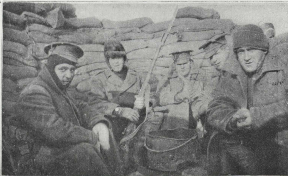
March, 1915. In First Line Trenches.
