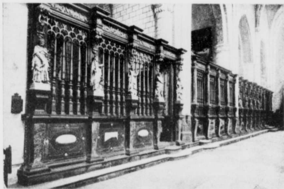
YPRES — ST MARTIN CHURCH MARBLE SCREEN WITH BRONZE BALUSTRADES
