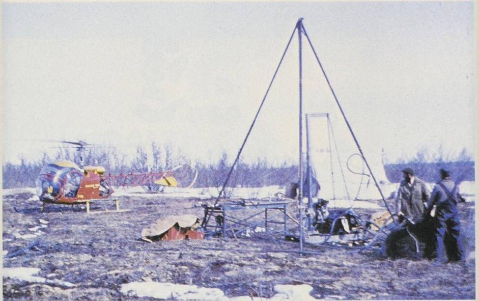
*Brown and Johnston often used a helicopter in the Aklavik survey (the search for Inuvik). To the right, a portable core drill used to sample the underlying permafrost.*
