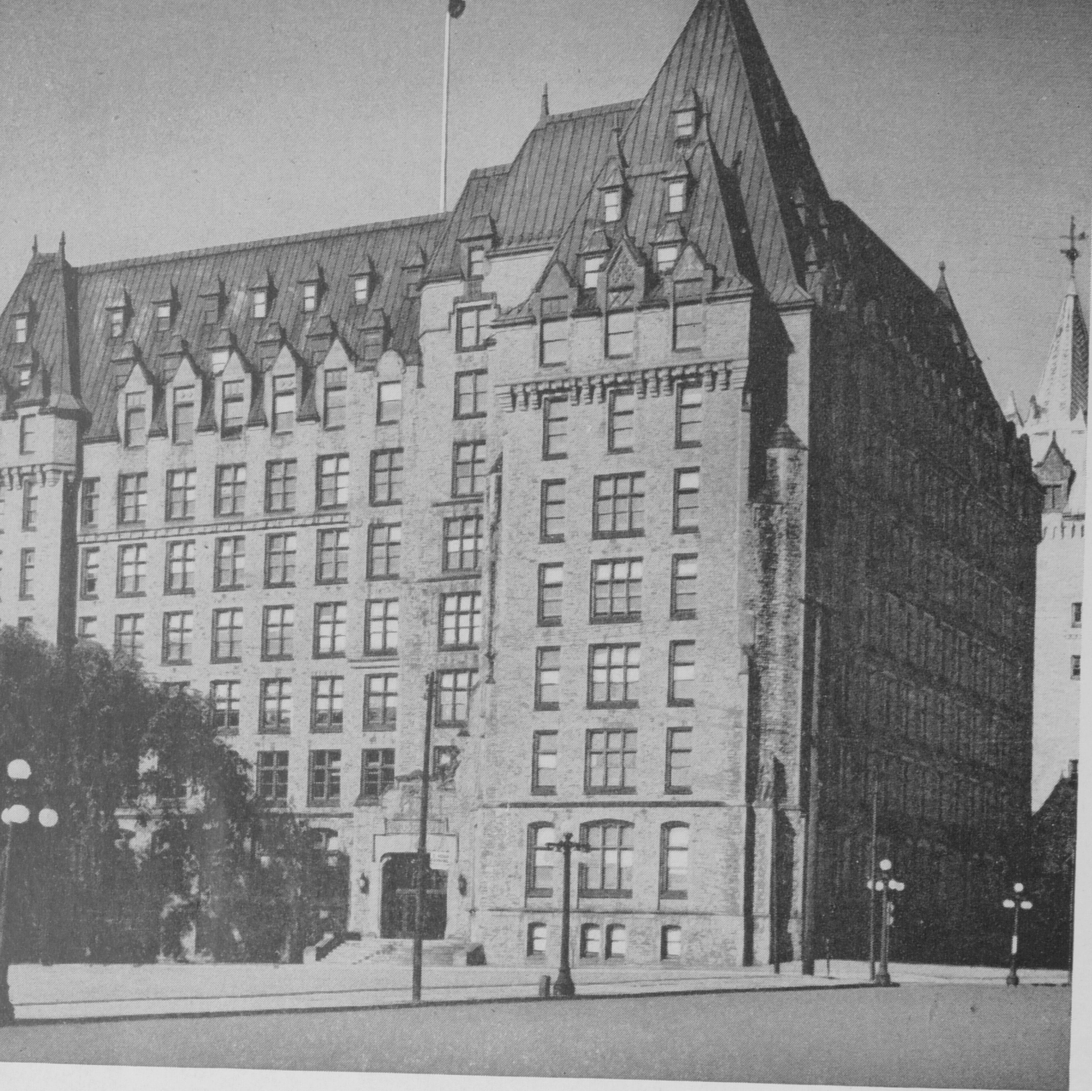
R.C.M.P. Headquarters, Justice Building, Ottawa. The Force's headquarters was moved to Ottawa from Regina in 1920.
