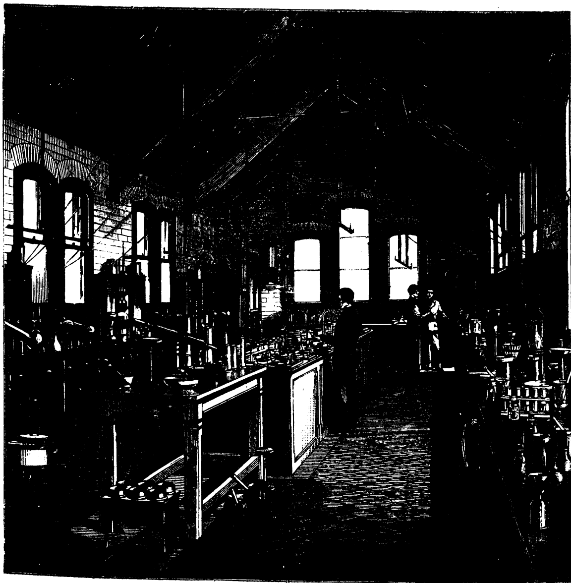
INTERIOR OF THE DYE HOUSE.
