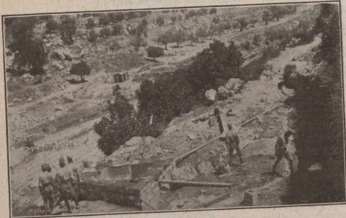
INTAKE, AIN ED DILBE AND WADI REIYA SPRINGS WATER SUPPLY
