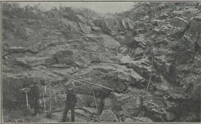
Open Cut at Bessemer.
