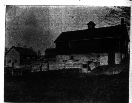
HENHOUSE AND PIGGERY, 16 x 20 FEET.—Wall, from foundation to peak, built with Thorold Cement, also floors. Walls 11 feet high at eave, 9 in.thick; also cement troughs.
