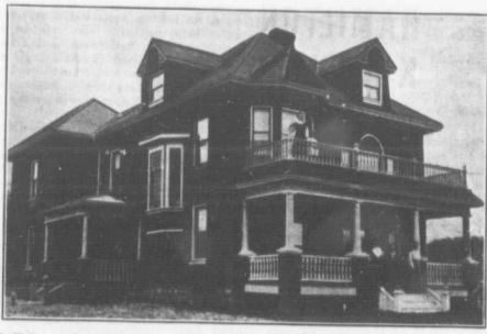
A Modern and up-to-date farm home owned by Mr. Oscar A. Waite, Brant Co., Ont. (See floor plan, page 16)
