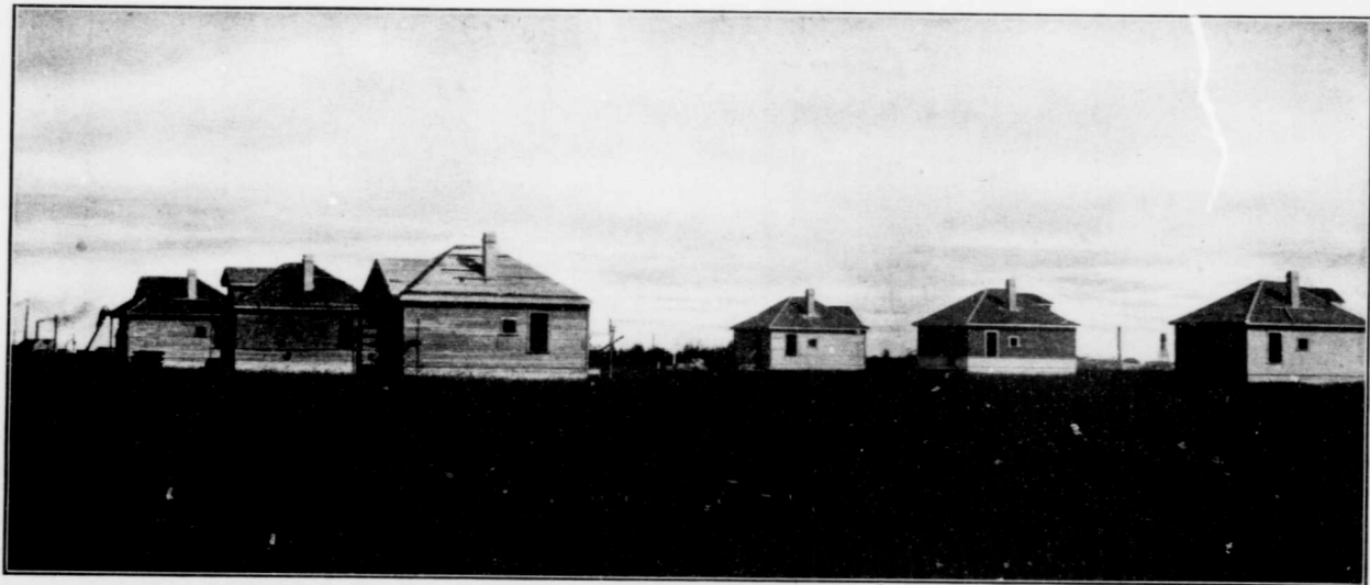
Six comfortable Cottages nearing completion, showing Dominion Tar and Chemical Works on left.
