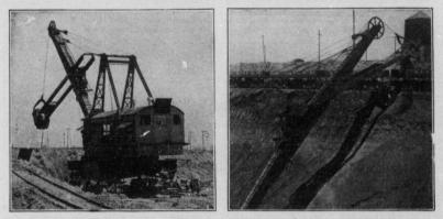
ONE OF THE SHOVELS WAS RIGGED TO LOAD CARS ON TRACKS 64 FEET ABOVE GRADE
