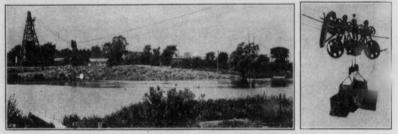
CABLEWAY EXCAVATOR AND NEAR VIEW OF GRAB BUCKET ON WELLAND RIVER SECTION
