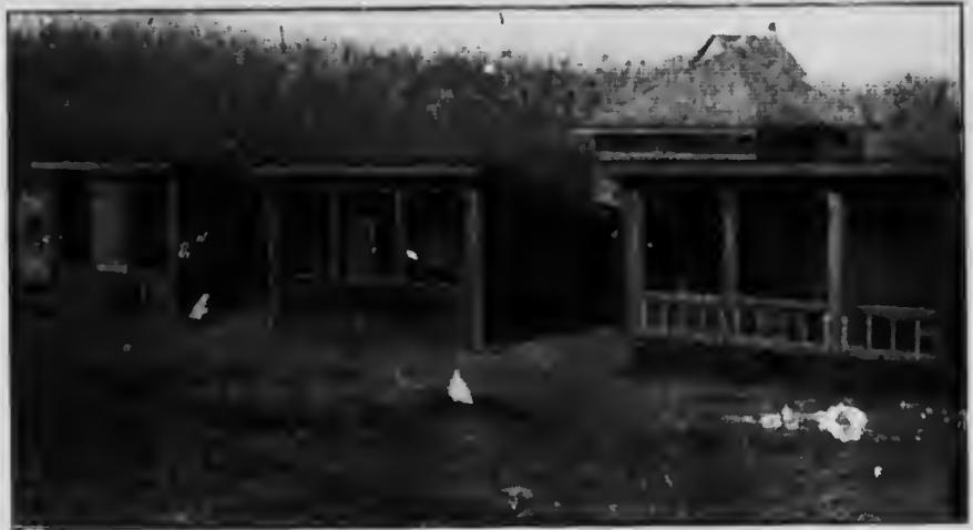
COTTON FRONT LAYING HOUSES USED AT INDIAN HEAD, SASK. These houses are 12' x 16' and on the level prairie can be moved with ease by a four horse team.
