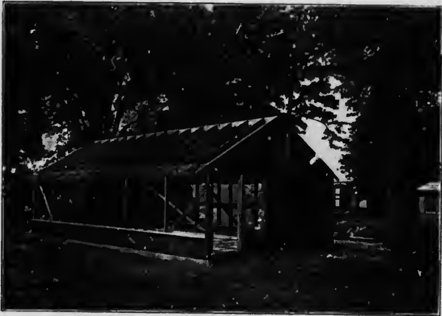
FRAME OF STRAW LOFT HOUSE.
