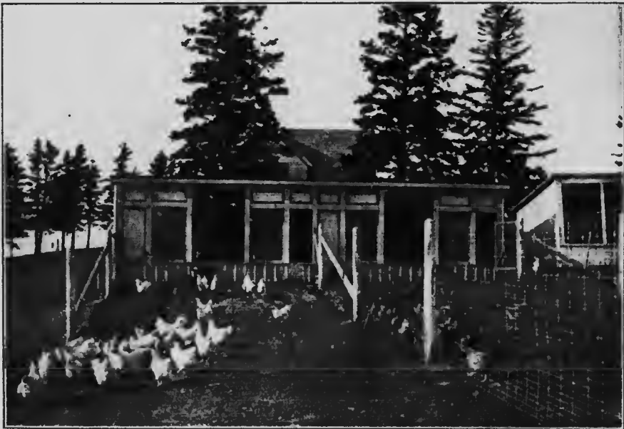
FARMERS' POULTRY HOUSE, SHED ROOF, NAPPAN, N. S. The openings shown in the front are cotton.
