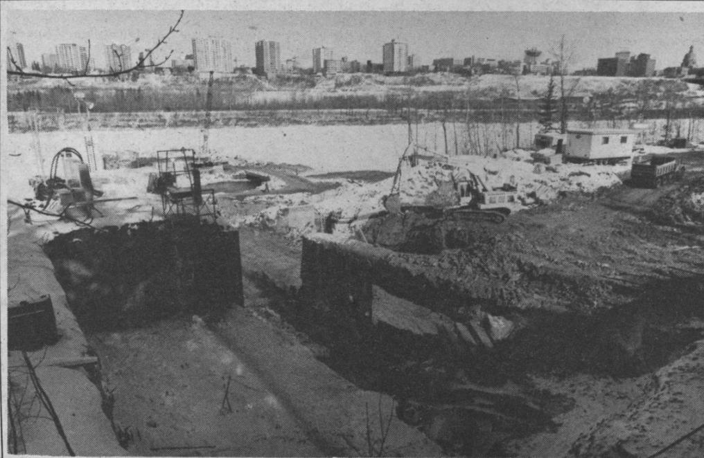
Chilled water anyone? Supplies should be plentiful when this addition to the U of A's cooling plant is completed in 1980/81. University buildings use chilled water for air conditioning.
