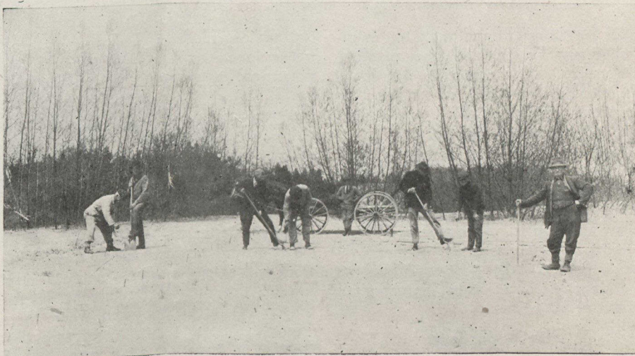
Blocking the sand dunes of Prince Edward County, Ontario, by planting trees. The planting gang is putting in willows and poplars. The willows in the background have attained their remarkable height in ten years.
