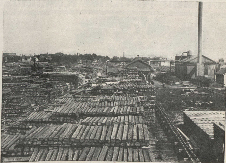
Thousands of railway track ties stacked in the yards of the Canada Creosoting Company, Trenton, Ont., awaiting the creosoting process that will almost double their endurance.
