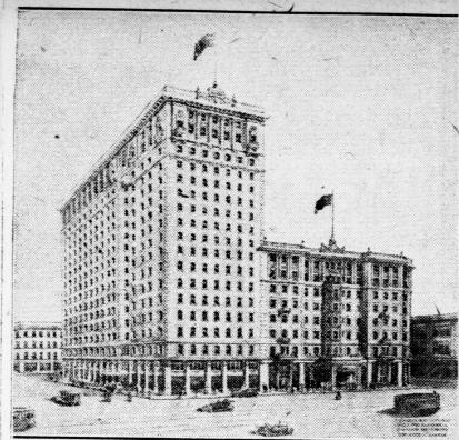
The above is a reproduction of a perspective drawing showing the King Edward Hotel, Toronto, as it will appear after the completion of the new eighteen-story addition, shown on the left of the cut, work on which is to start within the next few weeks. The new wing will contain 500 bedrooms, in addition to stores on the ground floor, and offices on the mezzanine. On the two upper floors will be the roof garden, with a seating capacity of 1,600 persons;
