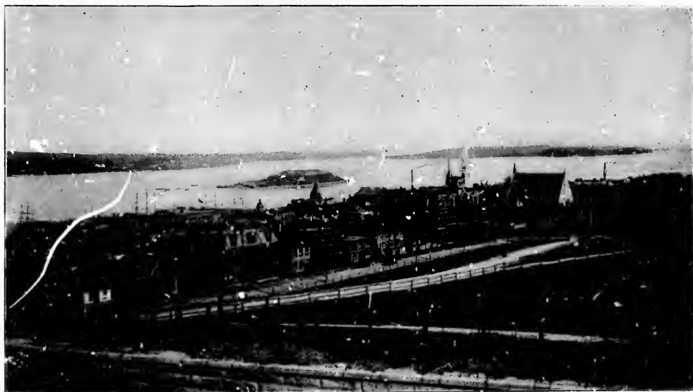
ENTRANCE TO HALIFAX HARBOR, N.S.
