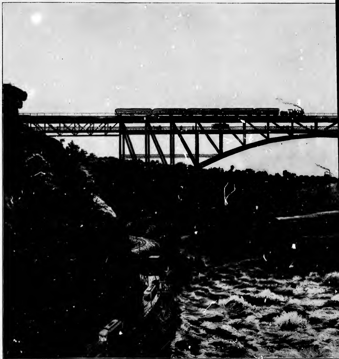
GRAND TRUNK NEW SINGLE ARCH, DOUBLE TRACK, STEEL BRIDGE OVER THE NIAGARA
