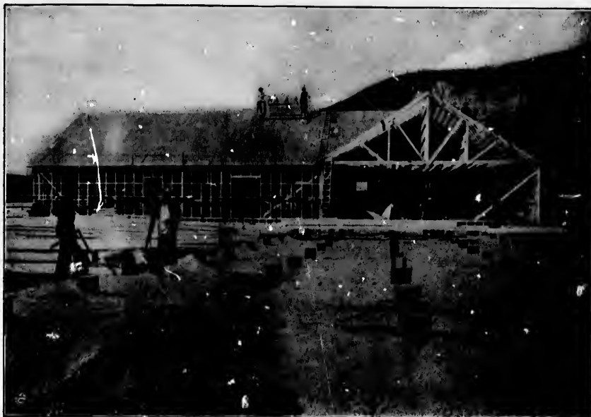
ALASKA COMMERCIAL CO.'S WAREHOUSE IN COURSE OF ERECTION AT DAWSON, JULY, 1897.
