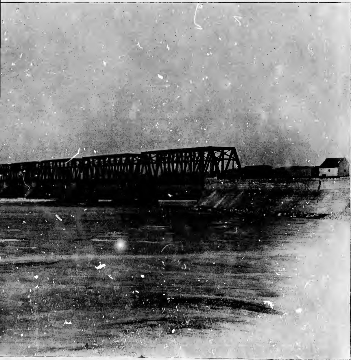
COMPLETED 1899, ACROSS THE ST. LAWRENCE RIVER AT MONTREAL, CANADA. racks, and double pedestrian and vehicle roadways. The superstructure replaced that of the Victoria Tubular Bridge erected 1854-59.
