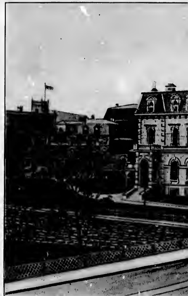
HEAD OFFICE, EASTERN TOWNSHIP RAILWAY
