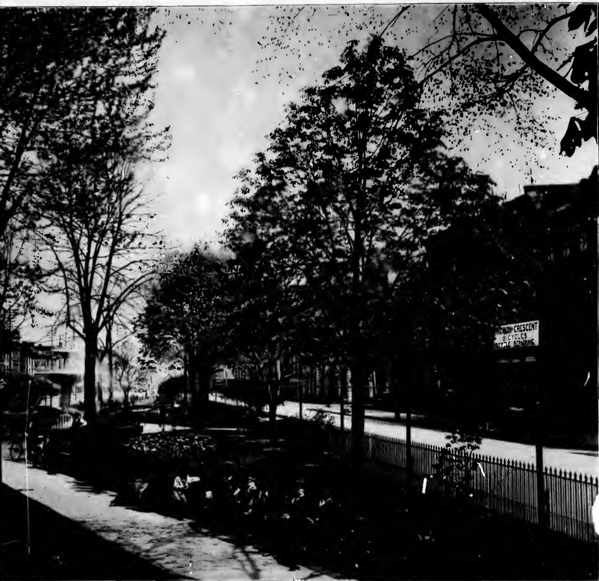
LOOKING EASTERLY FROM JAMES STREET, HAMILTON.
