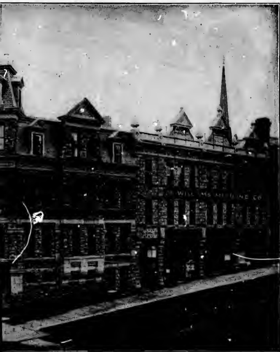
ORD BUILDING, BROCKVILLE, ONTARIO.
