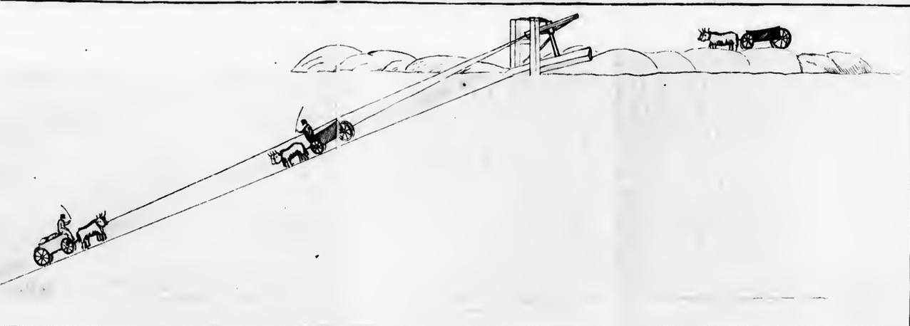
*Removing the Earth by means of machinery. — Scale 40 Feet to an Inch —*
