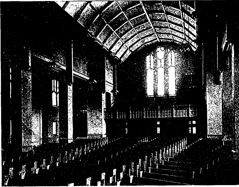
VIEW TOWARDS ENTRANCE, FIRST PRESBYTERIAN CHURCH, MONTREAL.
