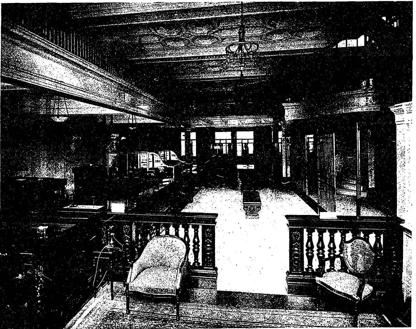
MAIN BANKING ROOM. TRUST AND GUARANTEE BUILDING, TORONTO.
