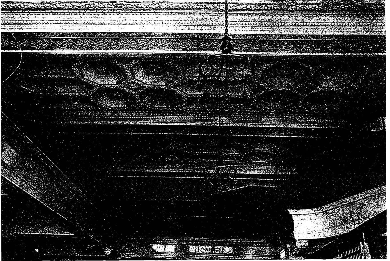
CEILING OF MAIN BANKING ROOM, TRUST AND GUARANTEE BUILDING, TORONTO.
