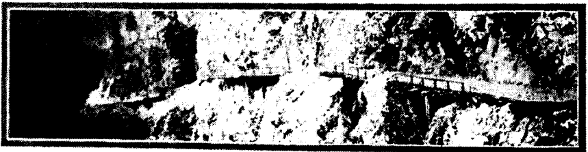
WHERE THEY PROPPED THE ROAD UP
