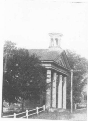
COURT HOUSE, KNOWLTON.
