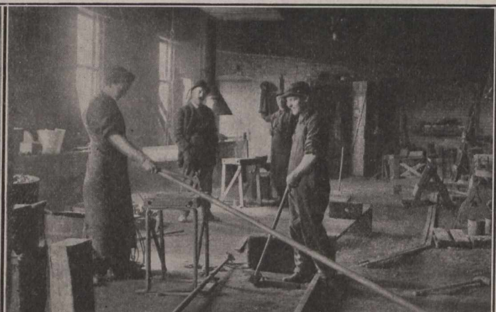
Fig. 5.—Interior of Blacksmith Shop, from the East.
