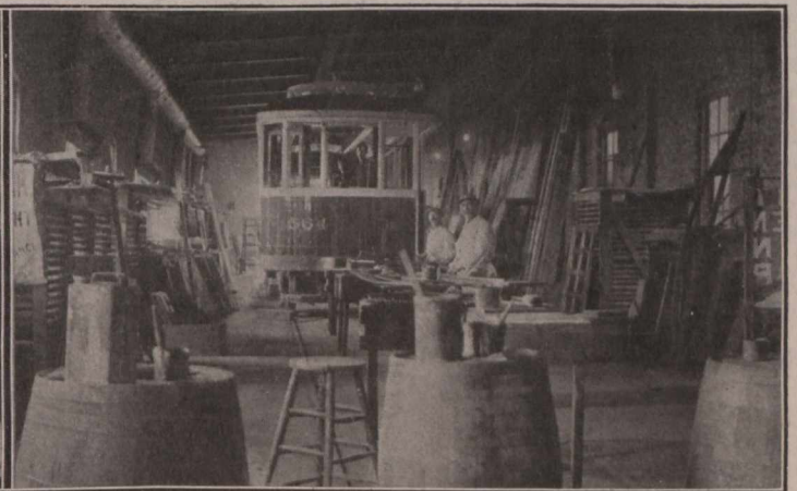
Fig. 3.—Interior of Paint Shop, from the West.
