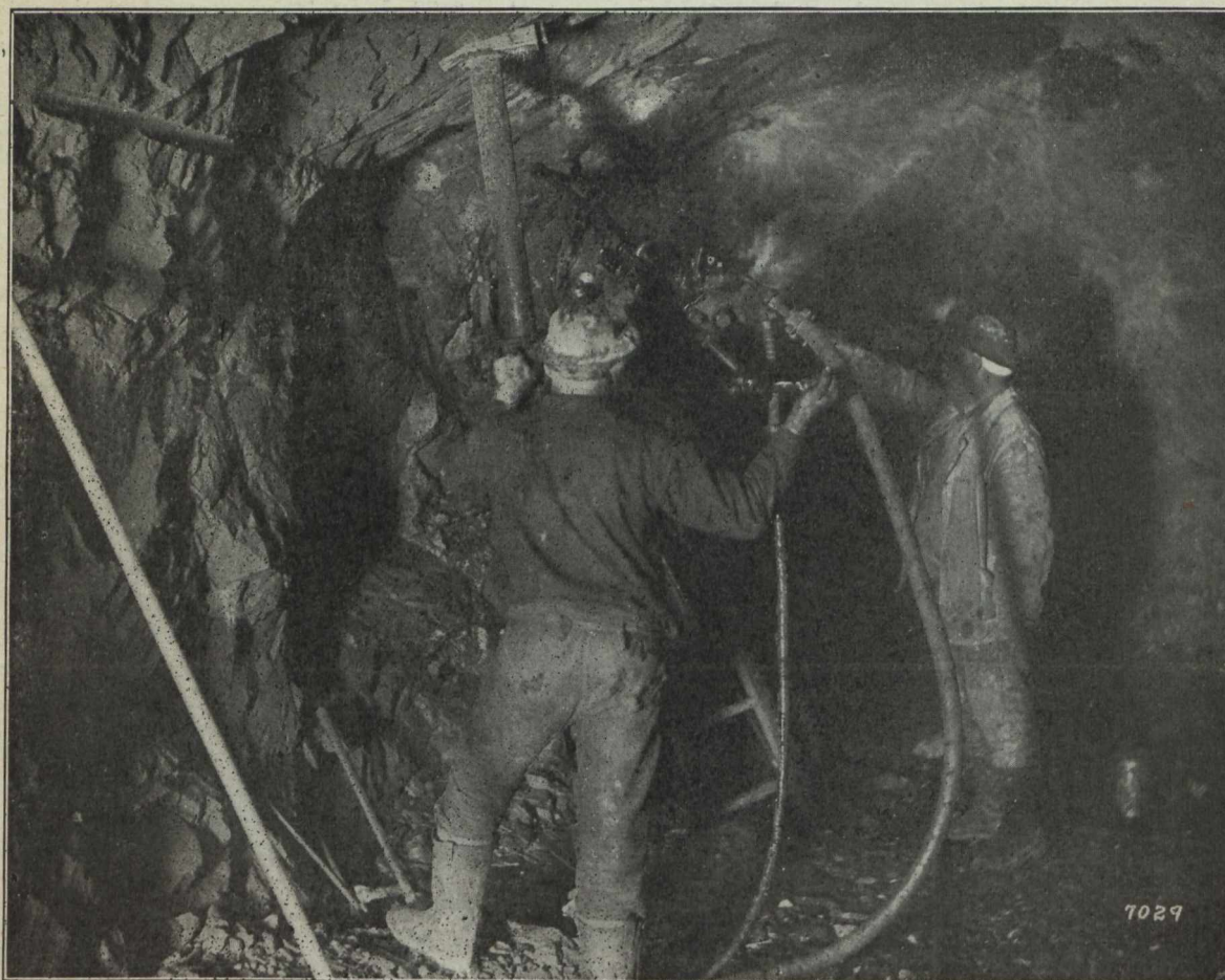
Drilling by Mounted Hammer Drill in a Lake Superior Copper Mine
