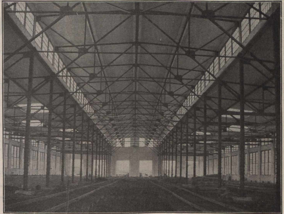
FREIGHT CAR REPAIR SHOP, INTERCOLONIAL RY., MONCTON, N.B.
