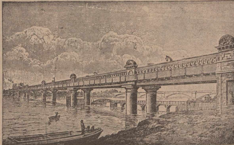
PUTNEY BRIDGE, OVER THE RIVER THAMES, LONDON.
