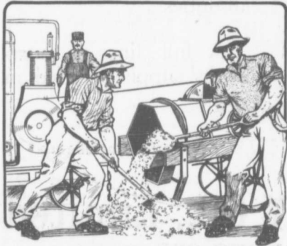
The Old Way of Handling Concrete.
