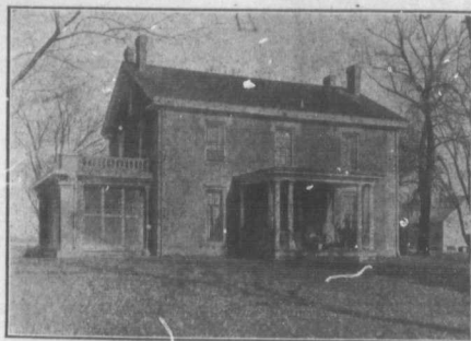
A Brick House Restored and Made Beautiful With Cement Stucco. This house was built on the grounds of the Agricultural College at Ames, Iowa, in 1882. Becoming dilapidated, the original brick was covered with stucco and a porch and screened veranda added as seen in the illustration. Many fine old Canadian farm homes now going into decay might be restored in the same manner.
