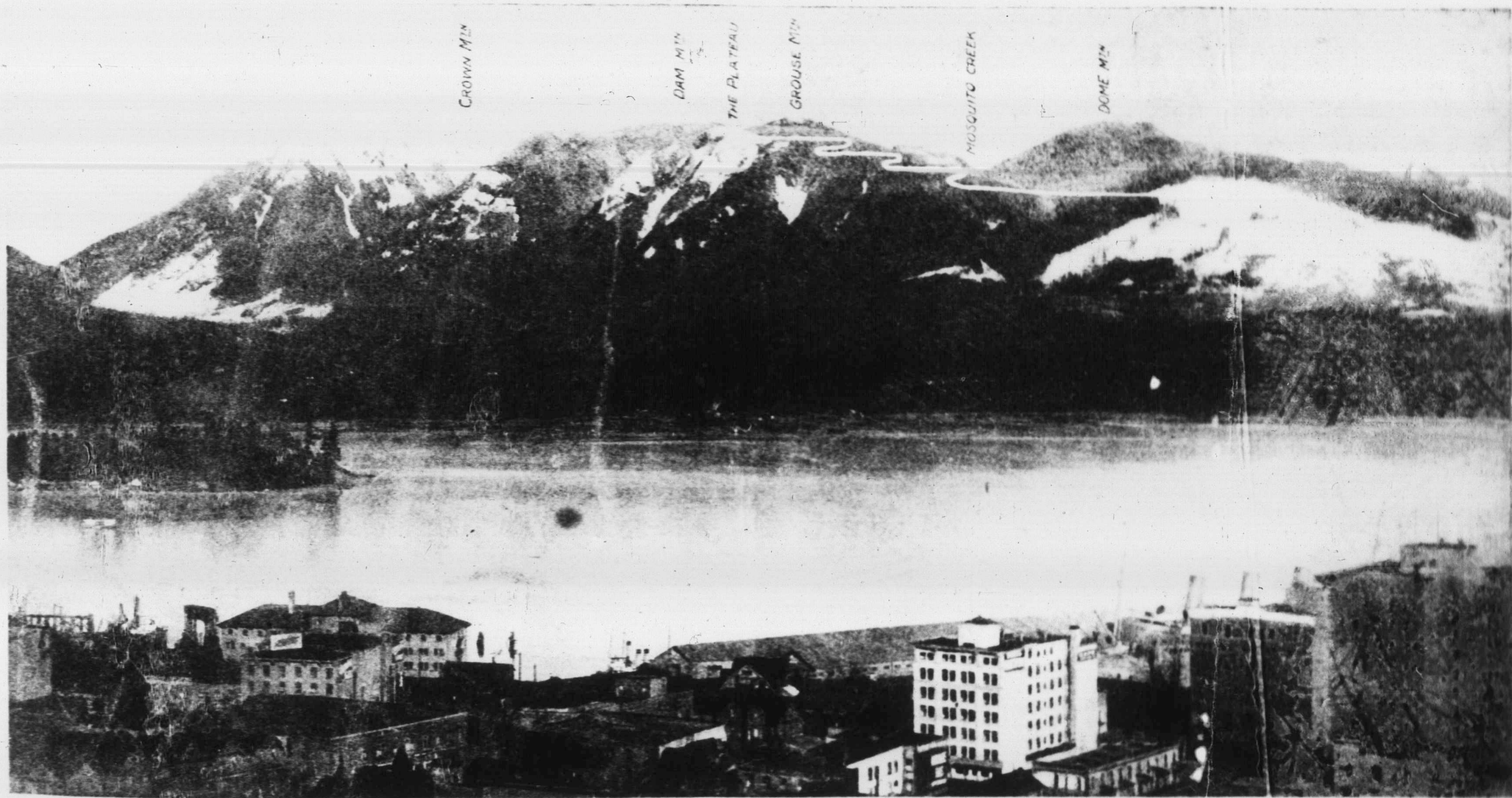
THE NEW NORTHERN TERMINAL OF THE PACIFIC HIGHWAY
