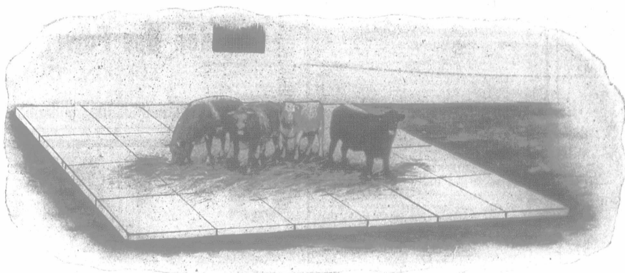
FEEDING FLOOR, 24x36 ft.—A feeding floor for sheep or cattle in the farmyard prevents loss and waste of hay, salt, grain, etc., and is easily cleaned. The illustration shows the general shape of a feeding floor which should be set an inch or two above the level of the farmyard, and also cast at a slight slope to allow water to run off.
