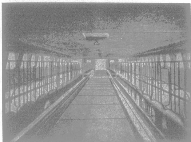
Cow Barn with running water in mangers, and central feeding passage, stalls and fixtures in gaspipe. Made of Portland Cement Concrete.
