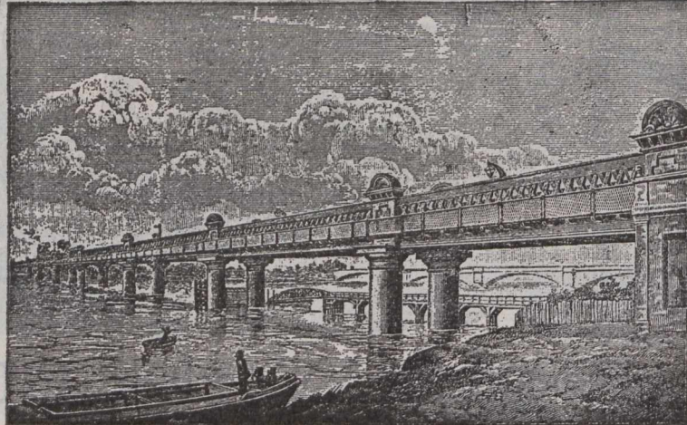
PUTNEY BRIDGE, OVER THE RIVER THAMES, LONDON.
