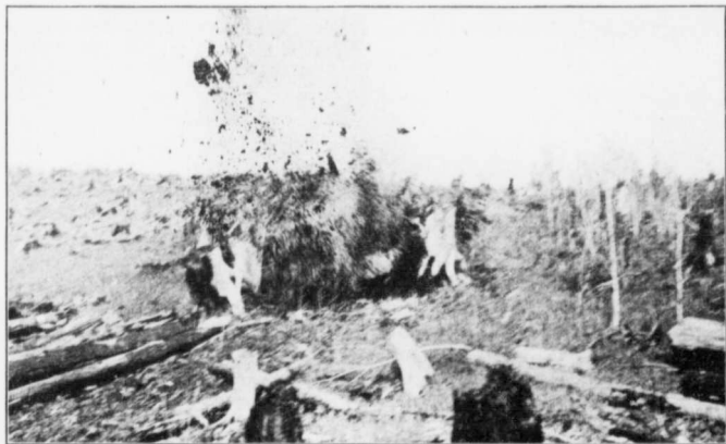
The same stump being blown up. Note the way it is being blown into pieces. This stump was removed for twenty cents.
