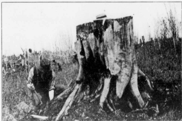
Placing a charge of dynamite under a large poplar stump.
