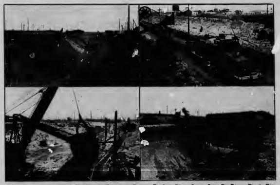
FOUR VIEWS OF ONE OF THE 8-YD. SHOVELS WORKING IN EARTH-TOP LEFT PHOTO SHOWS SOME RIP RAP IN PLACE-TOP RIGHT, TRAIN BEING LOADED AT STA. 846+81-BOTTOM LEFT, WORKING SOUTH OF THE WARASH R'Y-BOTTOM RIGHT, WORKING AGAINET & HIGH FACE AT STA. 346+81
