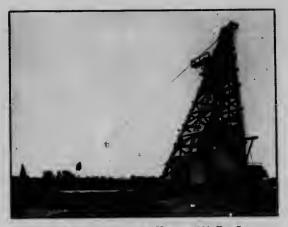
THE CABLEWAY EXCAVATOR HAS AN 800 FT. SPAN
