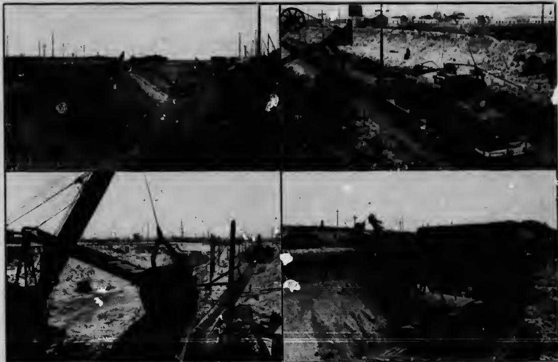
FOUR VIEWS OF ONE OF THE 8-YD. SHOVELS WORKING IN EARTH—TOP LEFT PHOTO SHOWS SOME RIP RAP IN PLACE—TOP RIGHT, TRAIN BEING LOADED AT STA. 346+81—BOTTOM LEFT, WORKING SOUTH OF THE WABASH R'Y—BOTTOM RIGHT, WORKING AGAINST A HIGH FACE AT STA. 346+81
