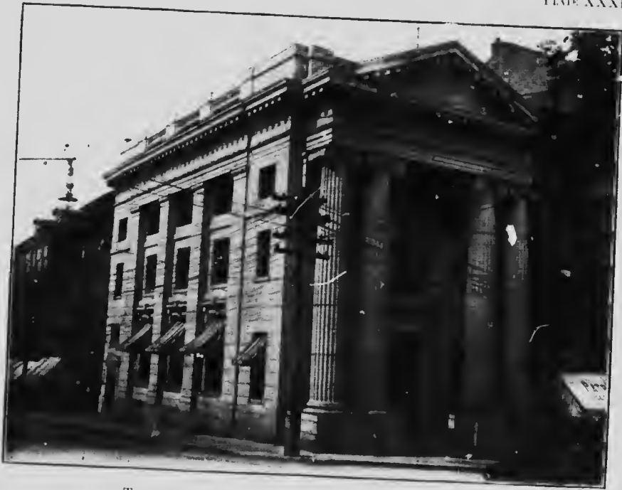
Terence Bay granite. Bank of Commerce, Halifax, N.S.
