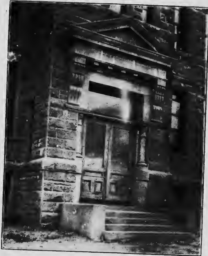
Miramichi sandstone. Door of Harkins academy, Newcastle, N.B.
