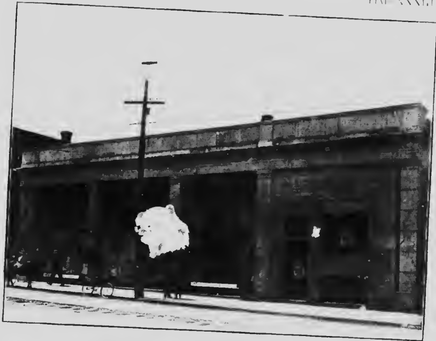
Halifax granite. Record building, Sydney, N.S.
