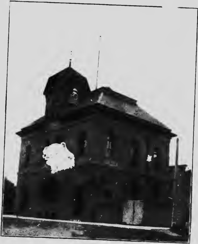
Grande Anse sandstone. Post-office, Bathurst, N.B.
