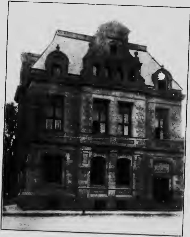
Miramichi sandstone. Post-office, Newcastle, N. B.
