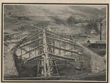
Sluicing an earth dam in Mexico—The earth in solution is discharged through the pipes, and the water runs off leaving the earth behind.
