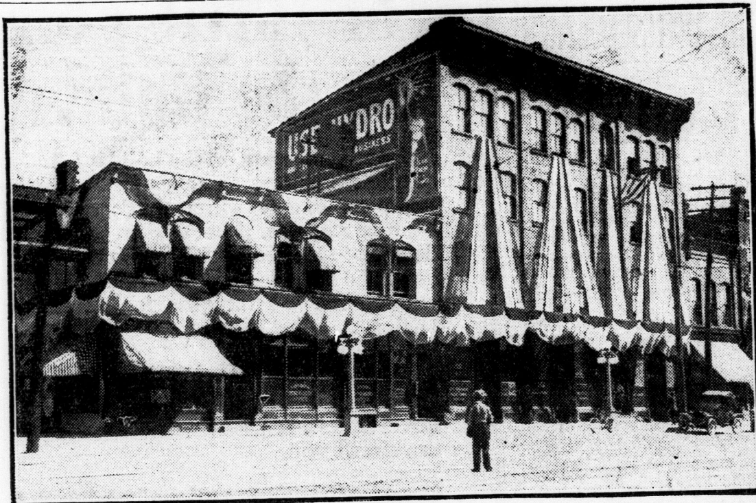
ORIGINAL SPENCER BLOCK IN DRESS UNIFORM. This is the Spencer block, purchased by the city in 1912 for $45,000, which will be disposed of as part of the plans which involve the transfer of federal square and Richmond street properties.
