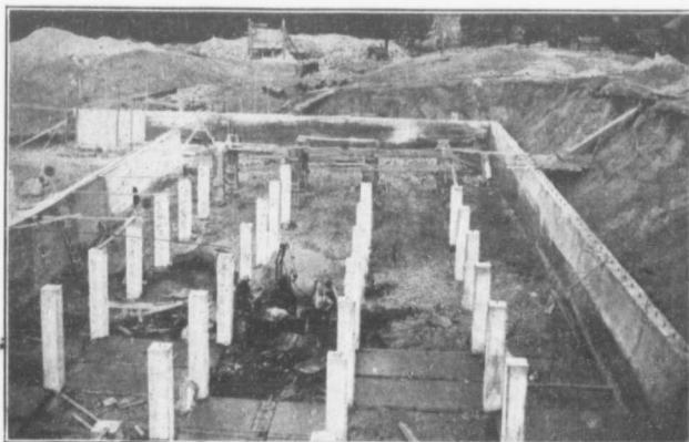
Filtration Plant Before Completion
