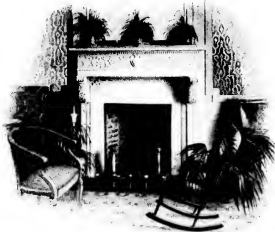
IN PLACE VIGER HOTEL
