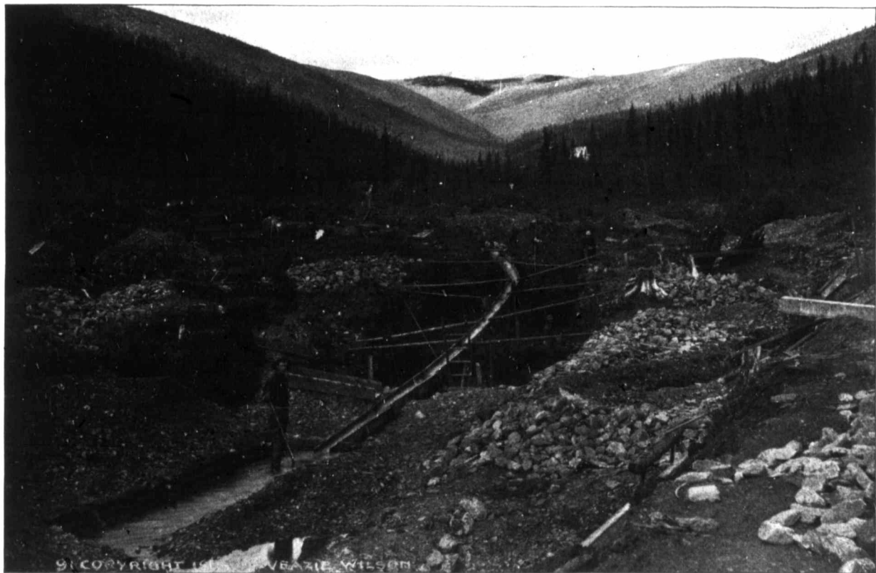
CLAIM FOUR ON MILLER CREEK. This shows the sluice, which is a long box with riffles. They are often joined in series and may extend several hundred feet.
