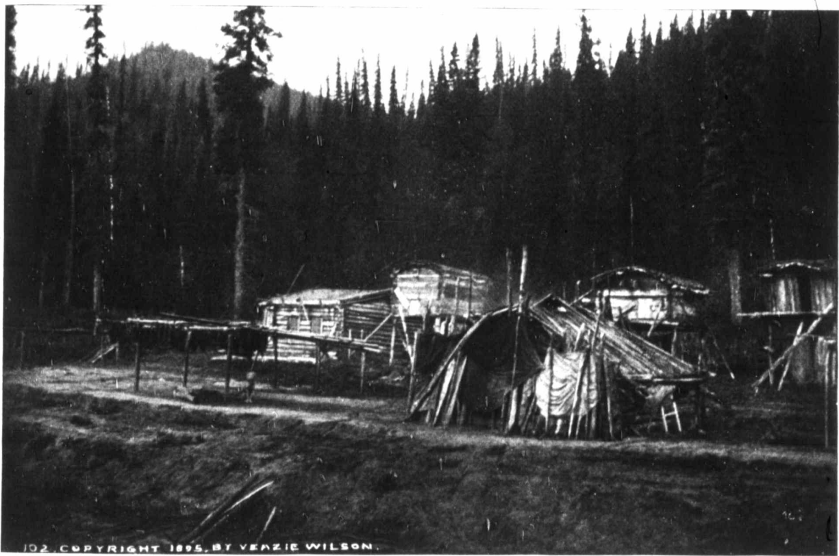
DRYING SALMON. Lower River. Showing caches. A cache is made by erecting a strong house upon posts twelve or fifteen feet above ground.
