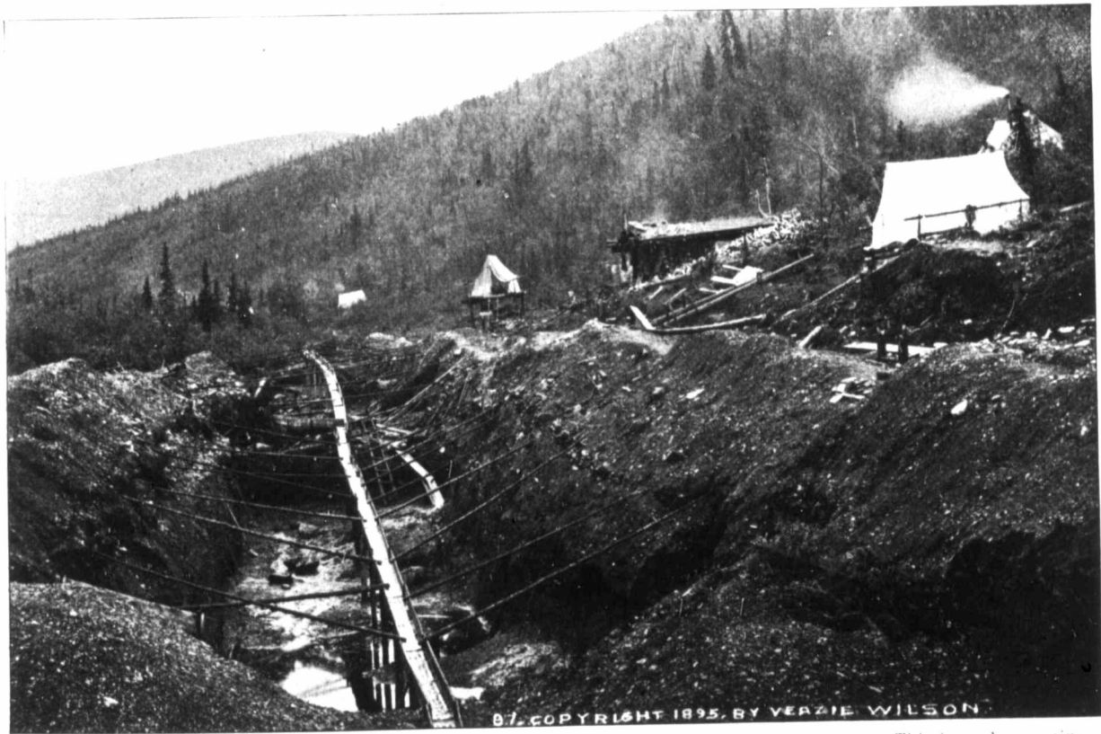
YOUNG AND BLANCHARD'S CLAIM AT MILLER CREEK. This shows the sluice boxes. (This is a placer mine. Placer is a Spanish word and means, literally, pleasure, that is, plenty of metal easily mined.)
