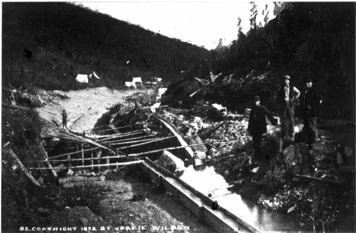
CLAIM THREE ON MILLER CREEK. $35,000 taken out; worked only thirty by one hundred feet, one clean-up being made of one thousand one hundred ounces.
