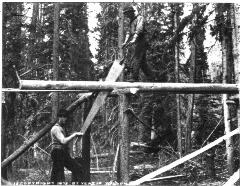
PRIMITIVE SAW MILL. Head of Lake Bennett. The timber has to be packed from where it is sawed to navigable water.
