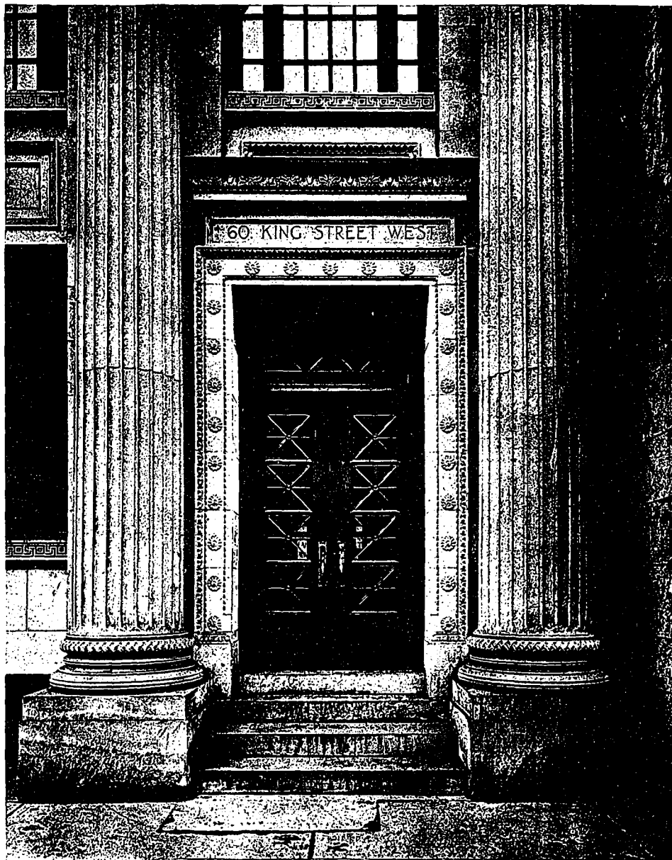
DETAIL OF ENTRANCE: BANKERS' BOND BUILDING, TORONTO.
