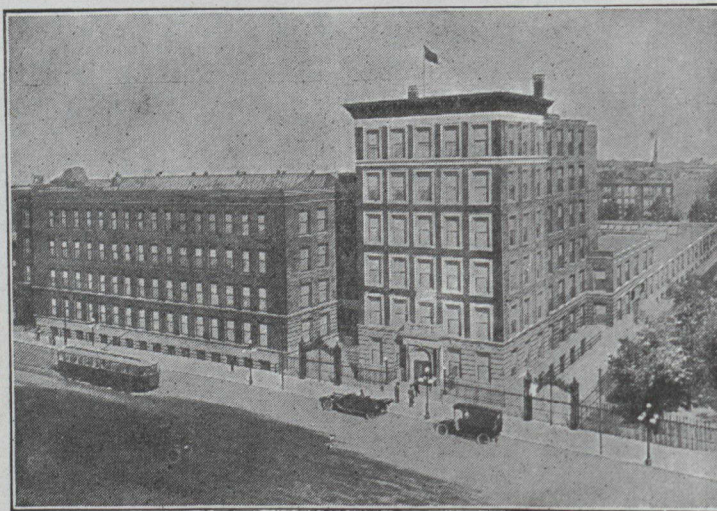
FIRE PROOF BUILDINGS
